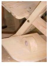
Check out the sandpaper patches. They were glued there to prevent the seat from slipping
